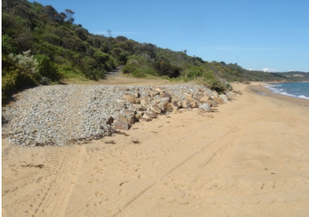
Unconsolidated material placed on landing in March 2015
